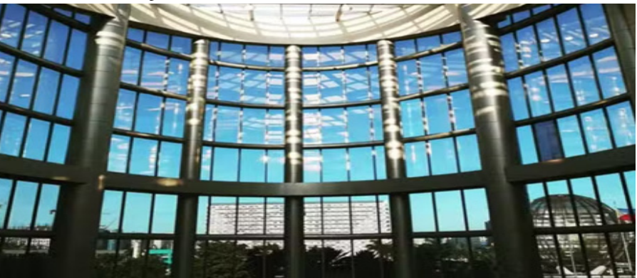
Natural light streams through the skylights of SM Supermalls, helping reduce electricity consumption while creating a bright, welcoming space.
