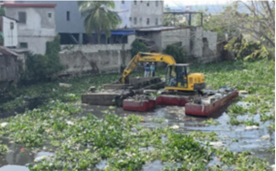
Alabang River, upstream of Cupang Bridge
